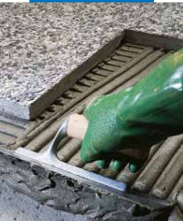
External installation of relief terrazzo "graniglie" tiles
