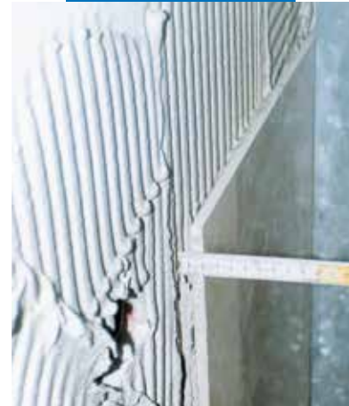
Thickly applied porcelain tiles on a wall
