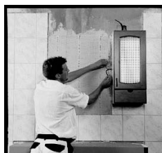
Cover with second layer to give smooth finish. Push connection tails into flex pipe.
