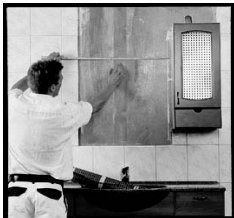
Measure the mirror and mark the area on the wall.
