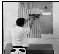
Cover the area with adhesive- check suitability of adhesive for mirrors.
